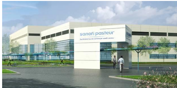
Dengue Facility Under Construction in Neuville, France
